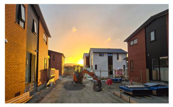
The development at 18–26 Strathmore Ave, Strathmore Park is a Kāinga Ora development that consists of 6x 2–bedroom units and two 4–bedroom standalone houses of timber frame construction built upon raised concrete slabs on blockwork upstands..
